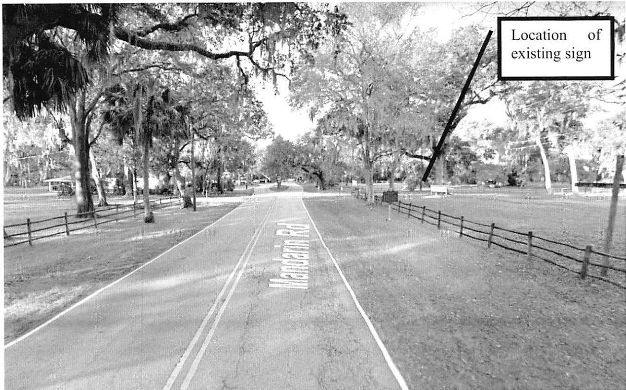
View looking west on Mandarin Road
